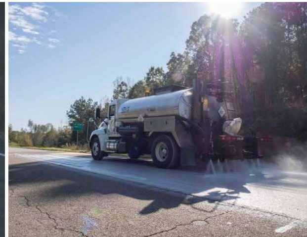
FIGURE 1 S3-A and S3-B application of spray-on rejuvenators.
