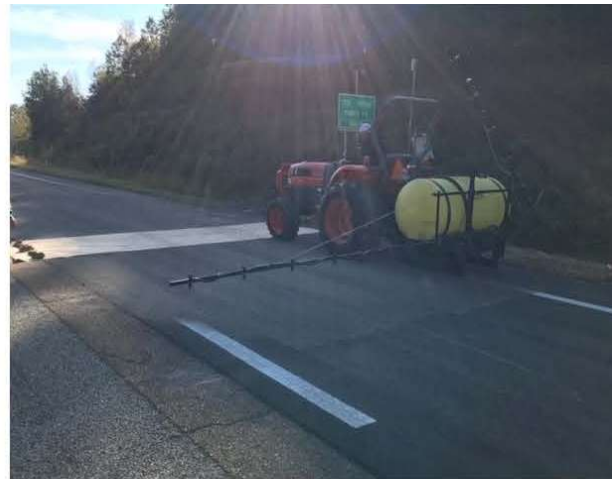
FIGURE 1 S3-A and S3-B application of spray-on rejuvenators.
